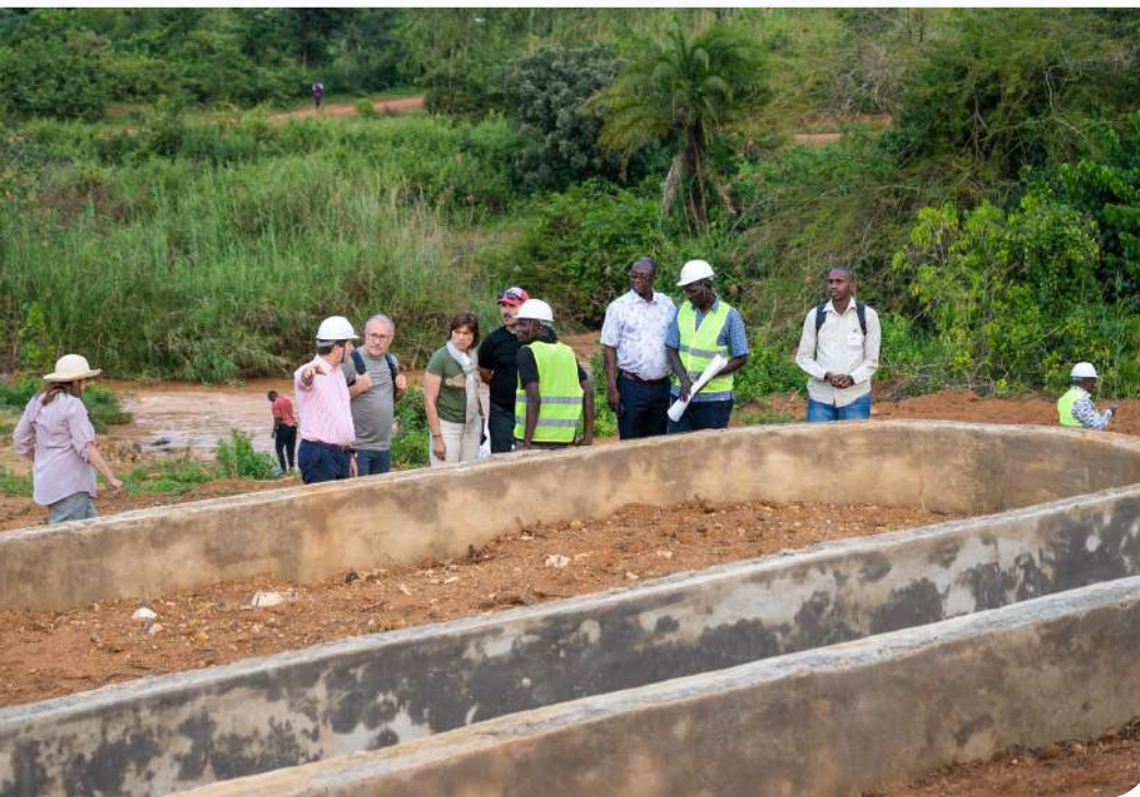
ECOHUB Engineer taking around INNOECOFOOD Consortium Partners during the visit to the Kenya ECOHUB on 2nd July 2025 at Ugunja, in Siaya County. The construction is still ongoing. Photo: Spirulina ponds under construction.
