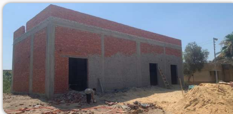
Ongoing construction fish processing using at Egypt ECOHUB.
