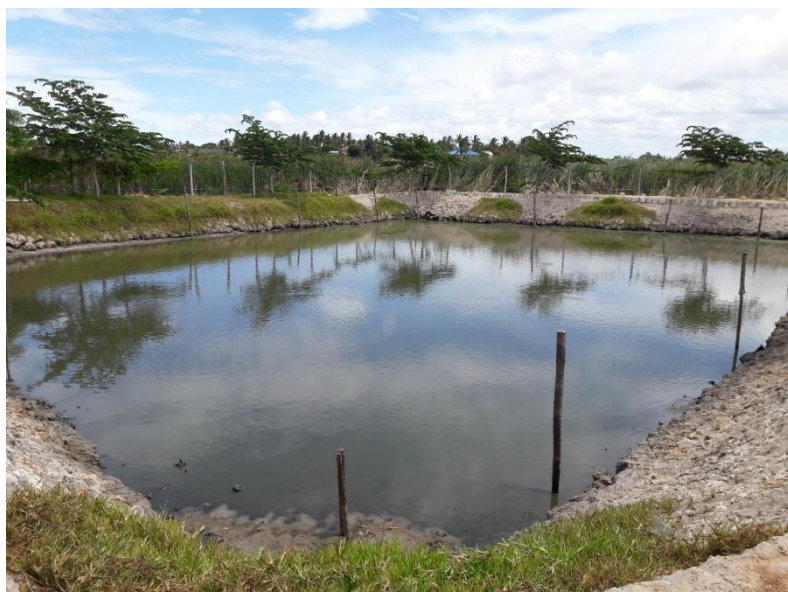
Figure 14. Example of semi-intensive fishpond system in Tanzania.
