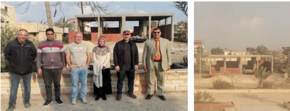
One of the facility building of ECOHUB in Egypt is under the construction in the CLAR.
